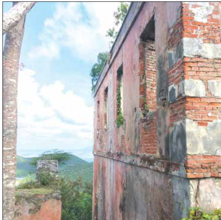
The America Hill Great House's red-tinted coral lime plaster facade stands out boldly among the island's natural blues and greens.
